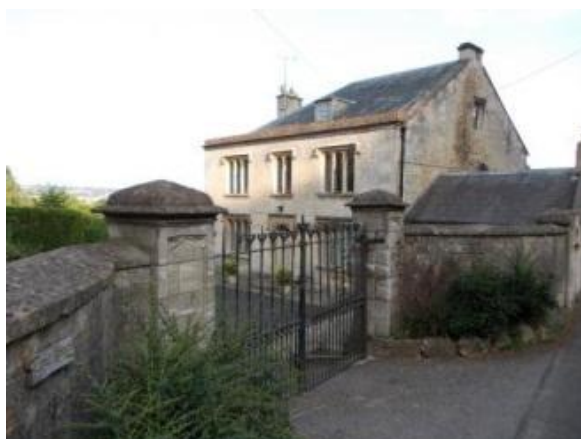
Long Court with Gateway and Wall
