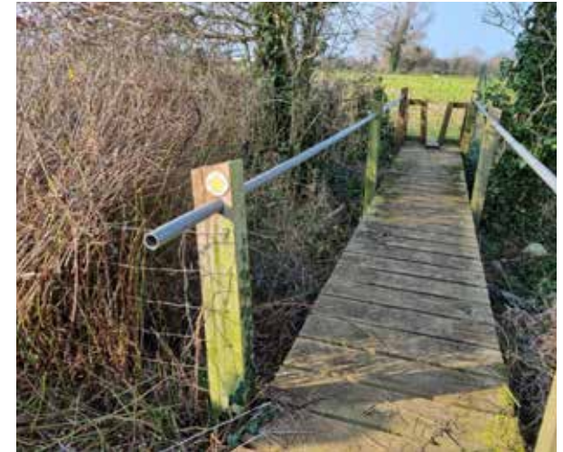
Recently cleared footpath bridge over ditch
