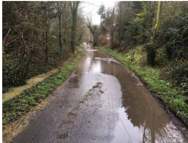
Flooding in Ryalls Lane - the ditches are full
