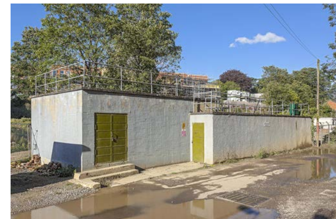
Severn Trent sewage pumping station – under review.
