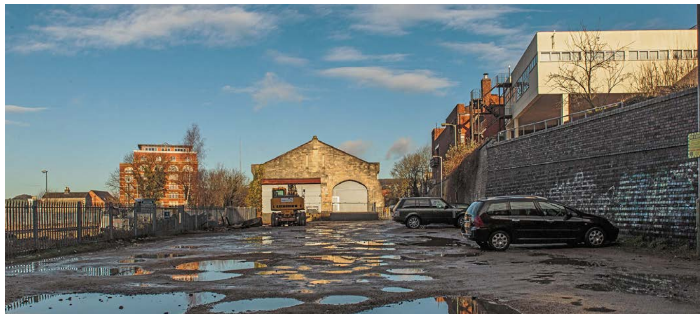
The Brunel Goods Shed east end.
