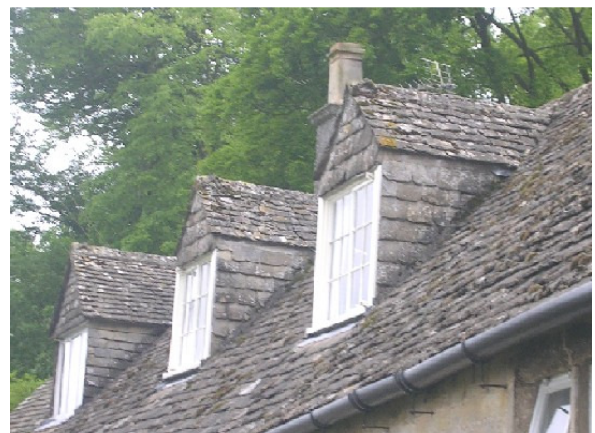
Below: Dormers on a Cotswold stone slate roof
