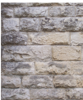
Left: Squared and coursed rubble stone wall
