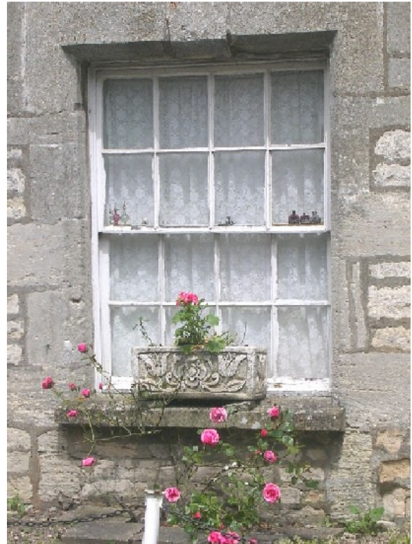
Above: A characteristic sash window on Bear House. Note the fine glazing bars and the lack of 'horns' on the top sash. This particular example is an 18 th century replacement for a doorway.
