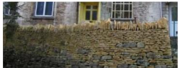
A recently constructed dry stone wall showing the tradition upright top row. Note that recycled stone has been combined with new stone
