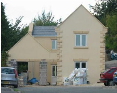
House under construction showing the combination of render with traditional features.
