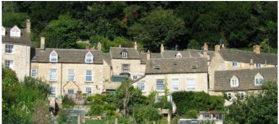
A range of cottages in Watledge demonstrating typical sash windows and dormers. Note the house in the middle that has modern skylight windows which are out of keeping with the character of the house and the area.
